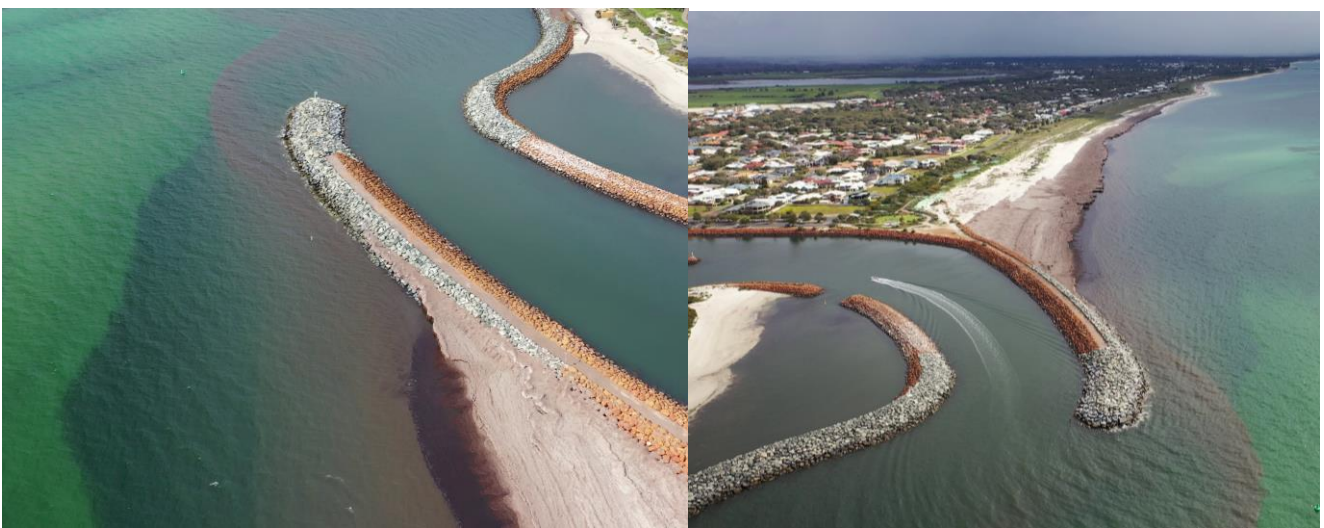
Figure 14: Natural bypassing of wrack along Western Breakwater during moderate westerly winds on 29 Sept 2019
